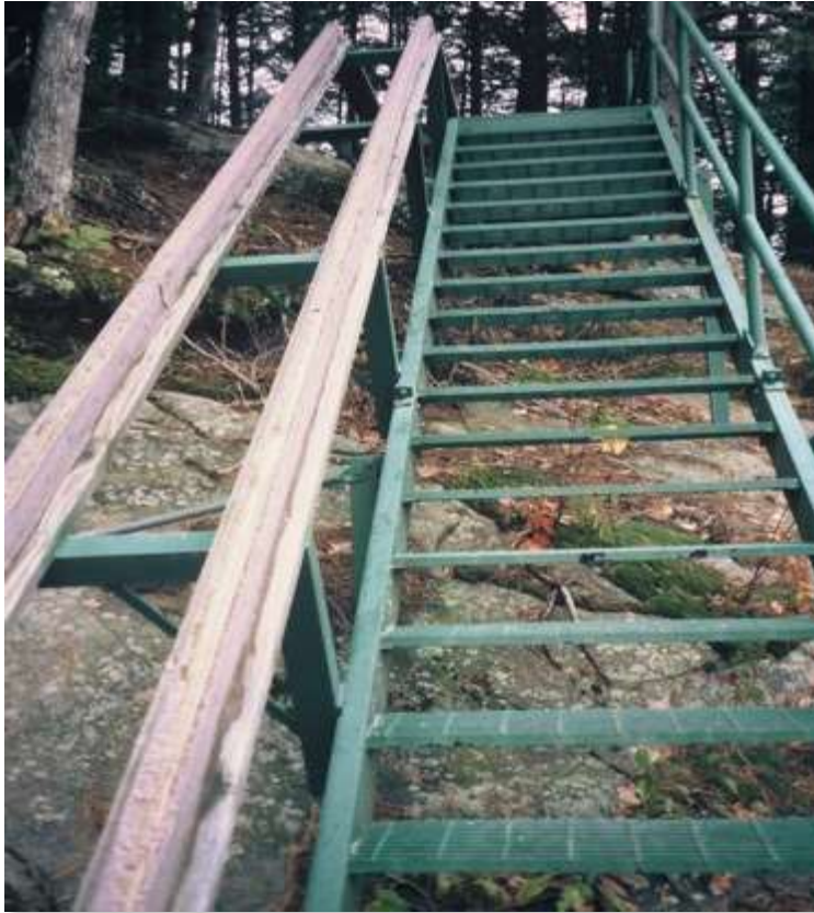
Steel canoe portage stairway with padded canoe slide in place to allow canoes/kayaks to be slid down to the river for launching
