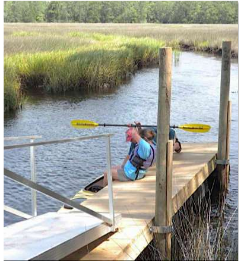
Treated timber piles on wooden dock
