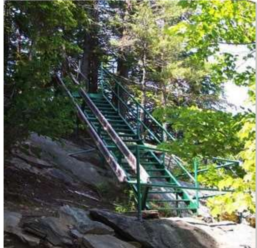
Steel canoe portage stairway with padded canoe slide in place to allow canoes/kayaks to be slid down to the river for launching
