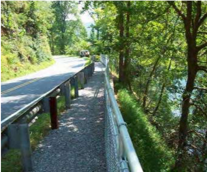
Cheoah River Roadside Portage Alcoa Power Generating Inc.
